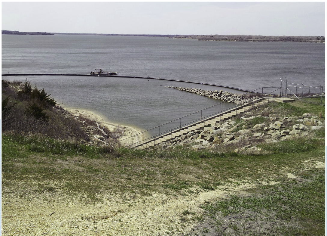
The barrier is held above the surface of the water by polystyrene flotation enclosed in an impervious hood. It extends to the reservoir bottom where the foot is held in place by chain ballast in a ballast pocket and by the forces acting on the barrier from water flow toward the dam.
