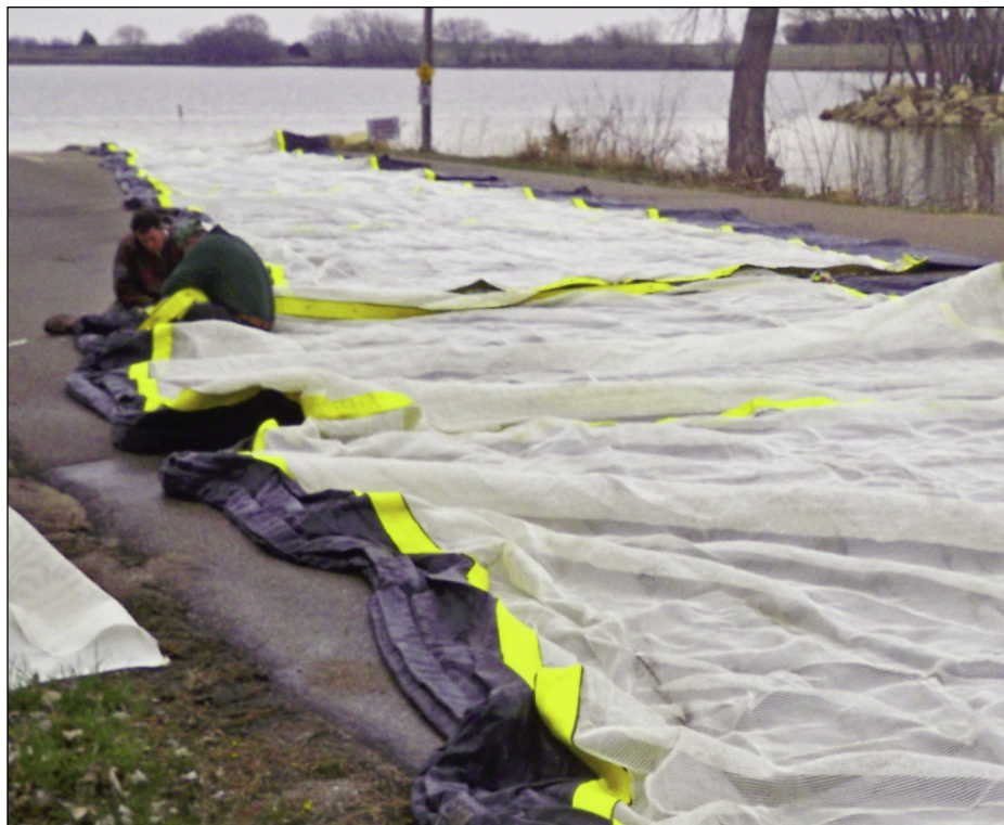
The middle section of the barrier consists of a coated nylon mesh with \frac{1}{4} inch holes. This mesh size was determined to be optimal for keeping the majority of the small fish in the reservoir while not allowing for fish to become impinged in the mesh.
